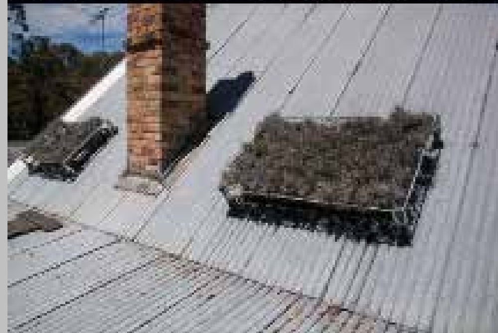
Above: the Tillandsia screens over and away from the skylights. Right: Tillandsia screen in flower.
