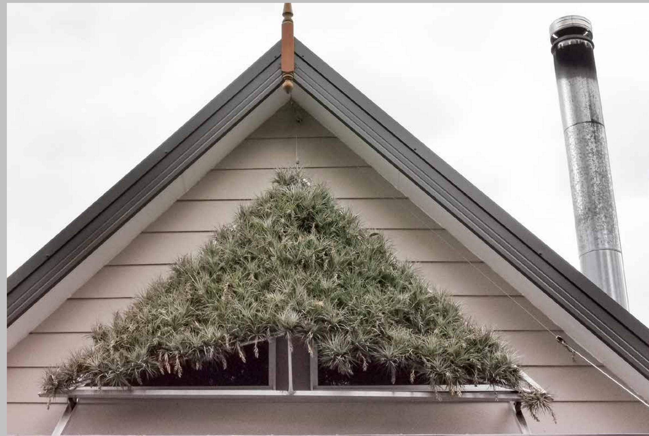
Photograph 2019 - Over three years the screen required no maintenance, and despite hot dry conditions, no plants died - the 2 photographs demonstrate the growth in the plants over this period. One plant far right bottom has slipped the mount but is still attached.
