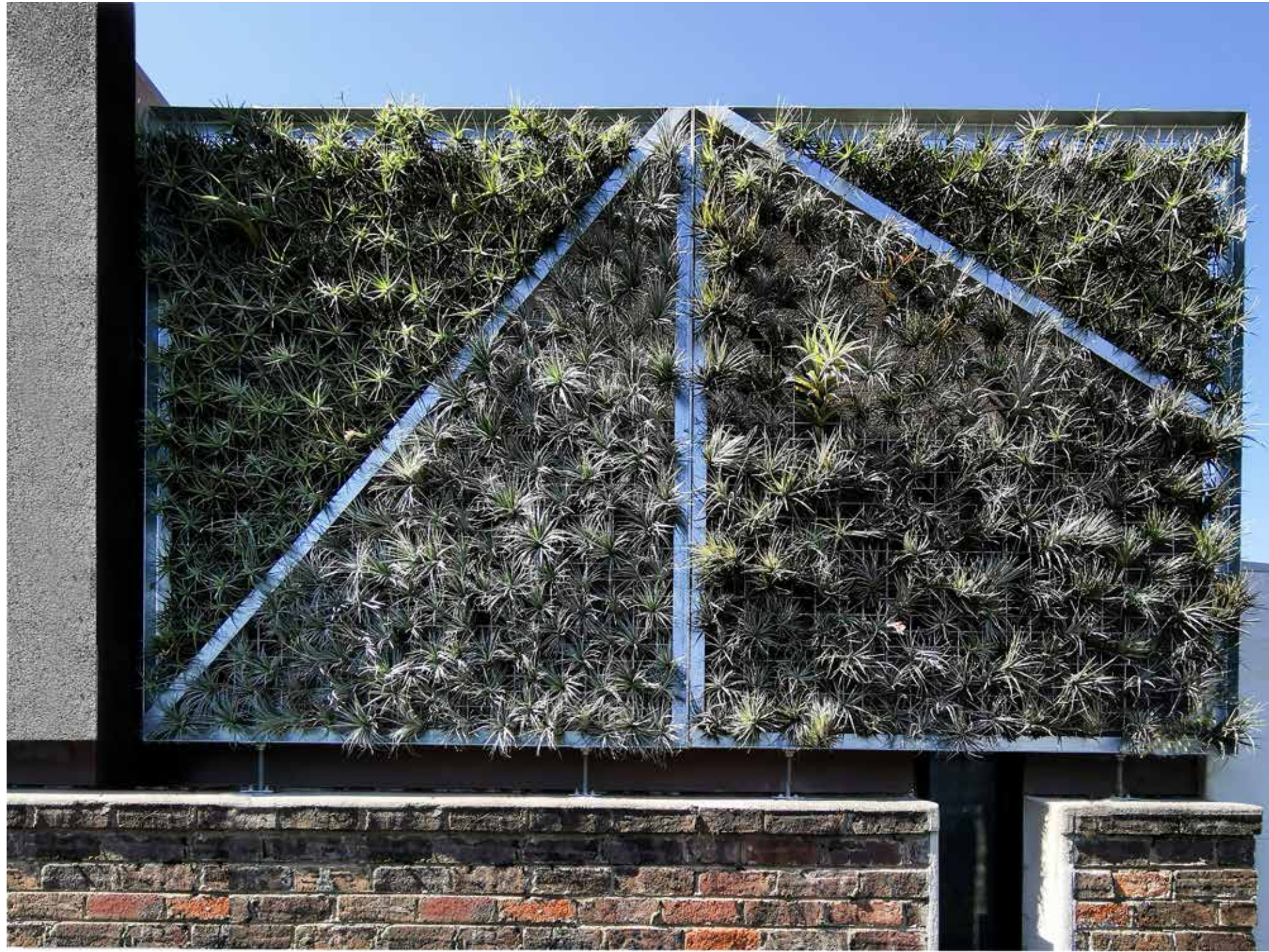
First two panels of Tillandsia screens installed March 2021..
