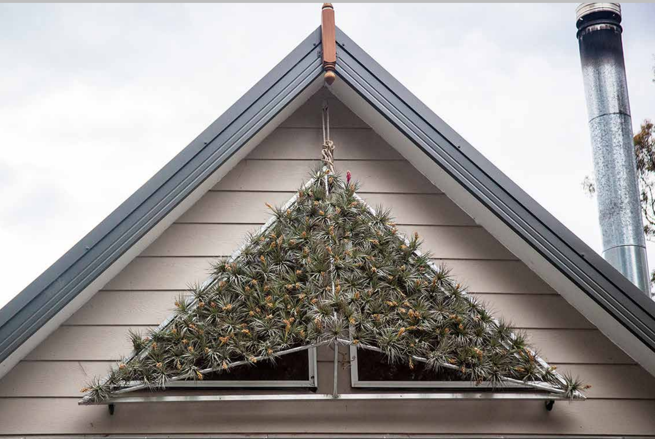
The screen is held in place during the installation before the wire cable and pulleys were installed. Notice how the screen is projected out from the wall at the bottom to allow light to enter the space. Photograph 2016
