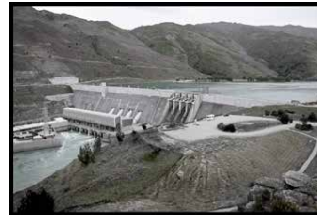
The Clyde Dam with Lake Dunstan - 2011
