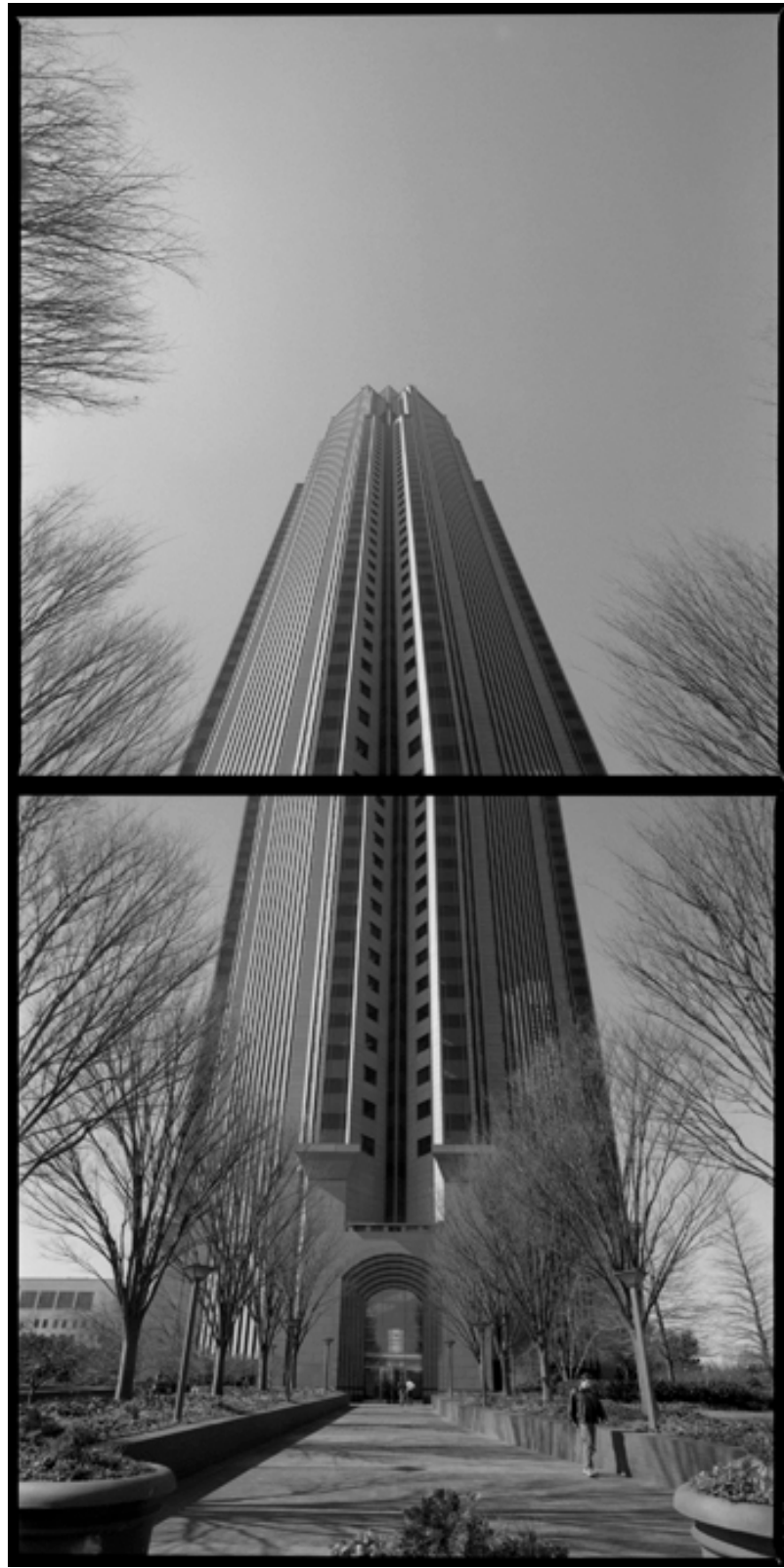
Bank of America building, Atlanta - USA 2005
