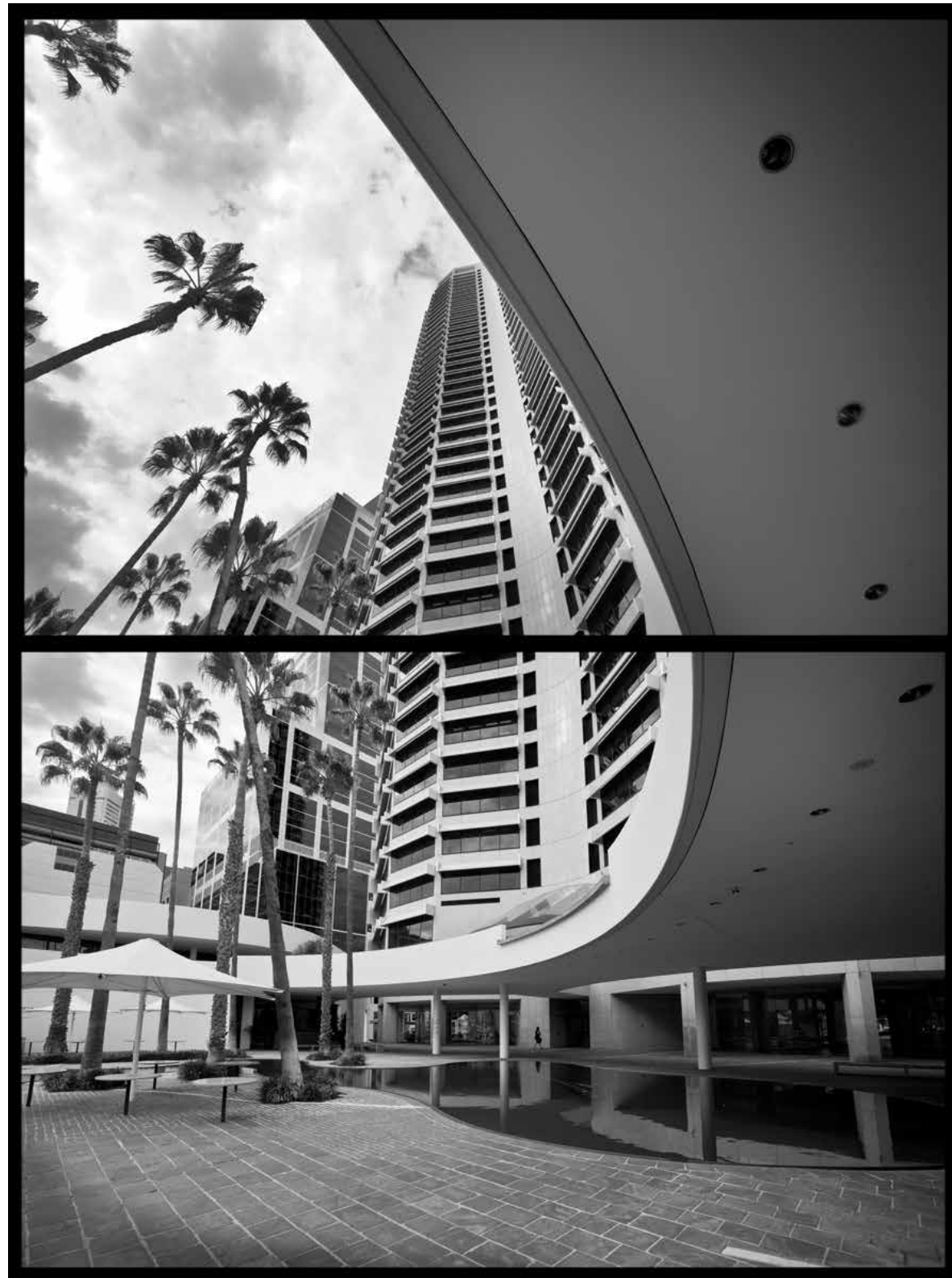
QV1 building , Milligan st , Hay St, Perth, Western Australia, 2012
