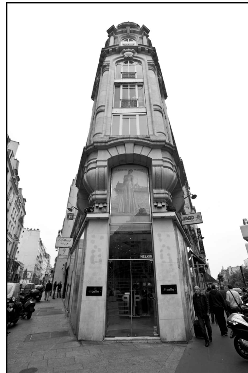
Rue Reaumur, Paris, France - 2010
