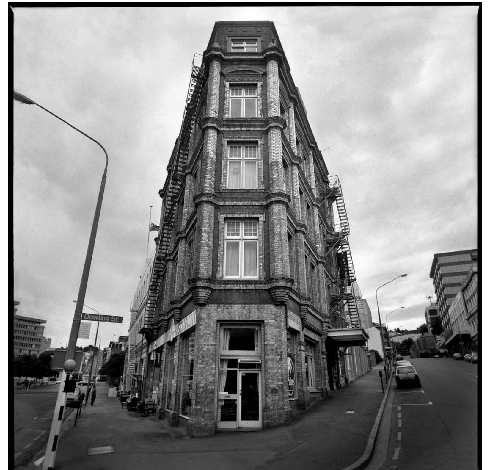
Imperial Building, Cr Dowling St & High st, Dunedin, New Zealand, 2002
