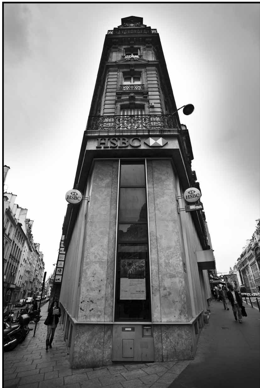
Rue Reaumur, Paris, France - 2010
