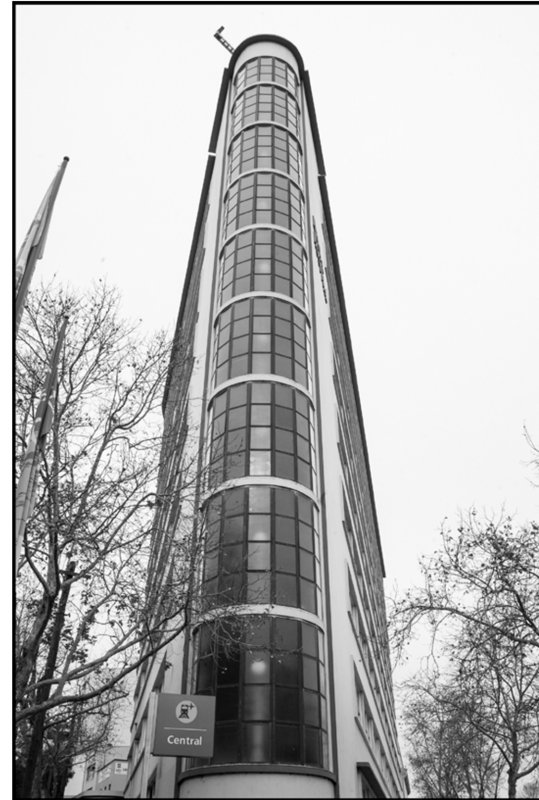
Cr Elizabeth and Chalmers St - Central Railway Station - Sydney Australia - 2008
